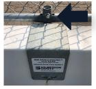
Tighten anchor bolt to barrier and set screw to fence panel
