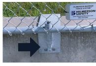
2 Set Side Saddle Bracket<sup>™</sup> and fence panel onto barrier
